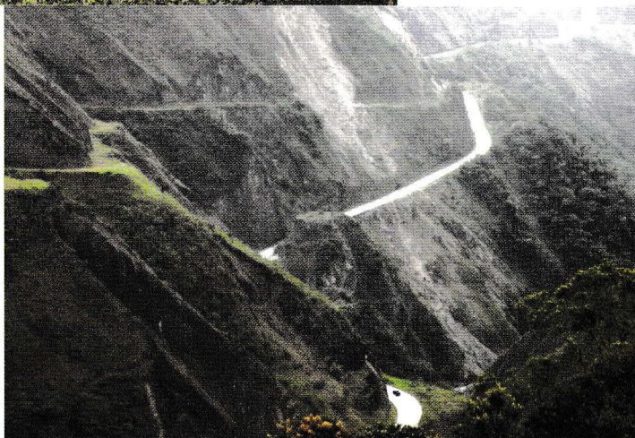
FIG. 2 B. Old and New Road between Loja and Zamora in the upper part of San Francisco valley with huge landslides, view to the east (ca. 2200 m a.s.l., photo: SWBr 12. 10. 2004).
